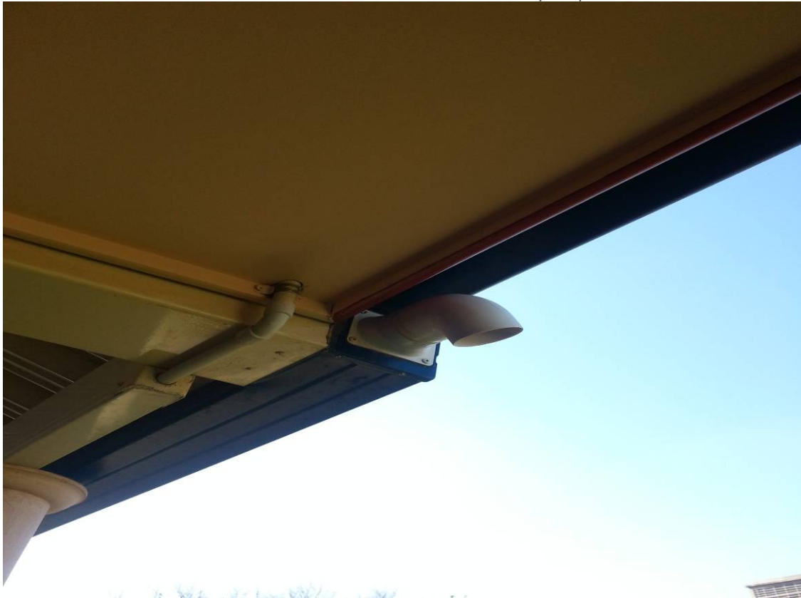
Photo 3: Downpipe opening to the pergola.
